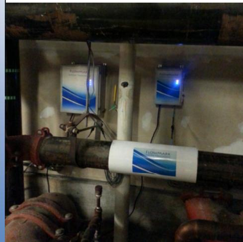
Mark-III installed on 6" pipe.
