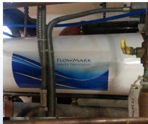
MK-IV installed on 10" pipe
