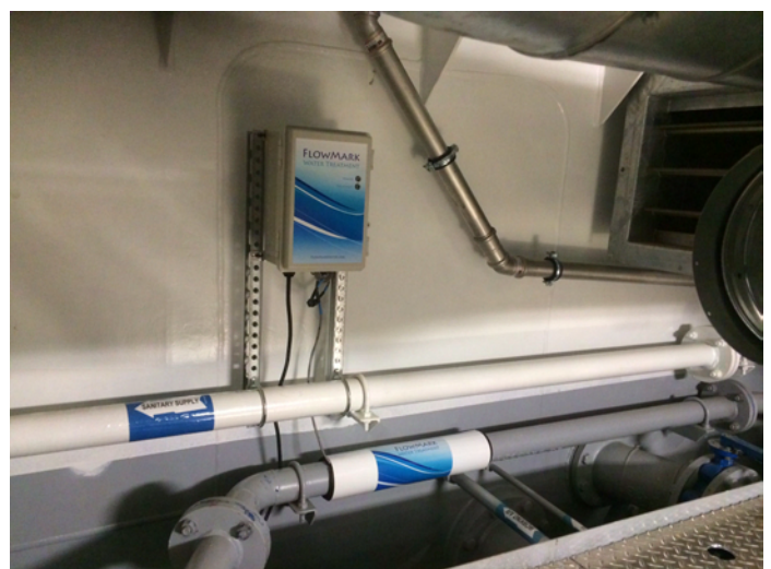
Two FlowMark model Mark-III systems installed on two new Fjord Line Ships
