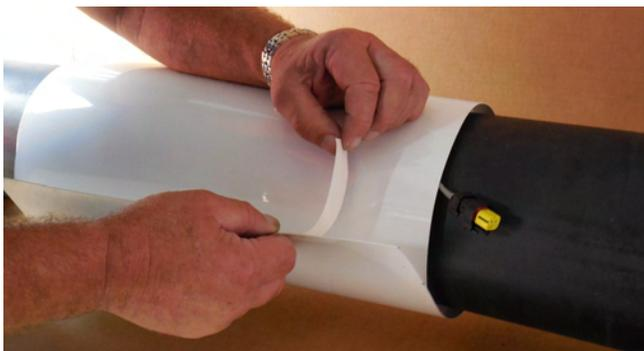
Remove adhesive strip and seal cover tightly.
