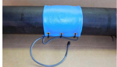
Install Treatment Pads Opposing Each Other with labels "To Pipe" facing the pipe.
