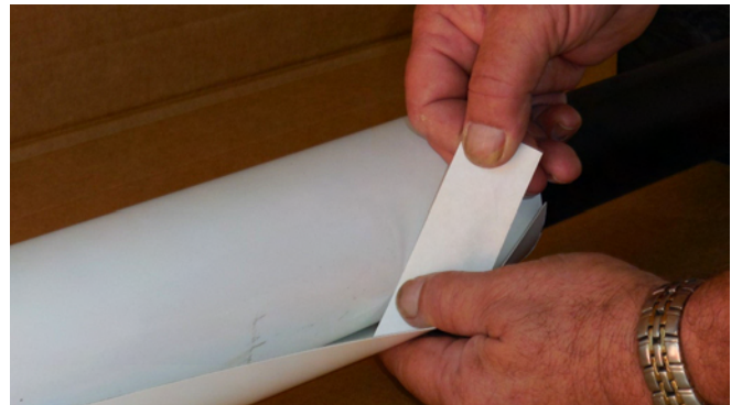
Tighten Pipe Cover for Snug Fit, Remove Tape and then Seal
